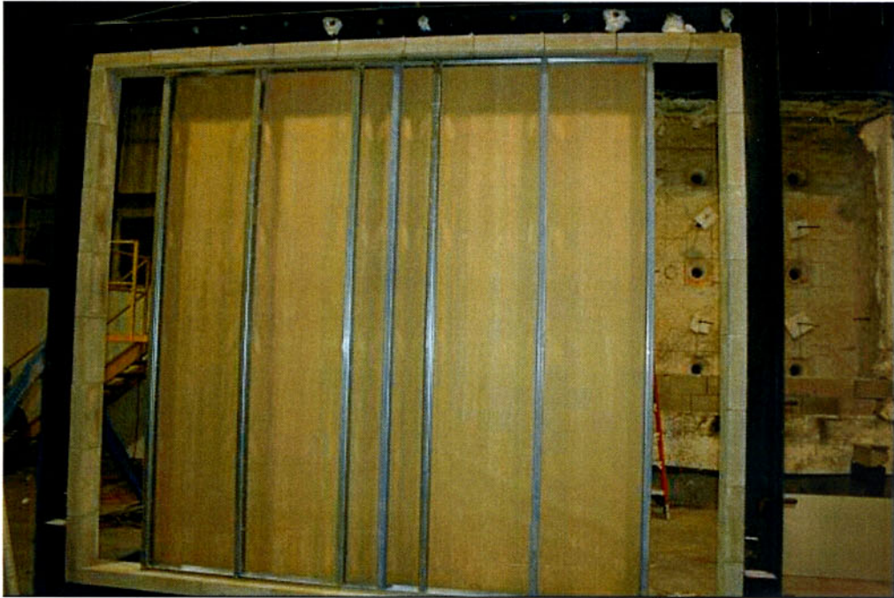
Figure B-1. Wall Construction in Progress.
