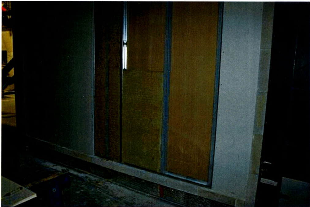
Figure B-2. Wall Construction With Insulation Boards Being Installed.
