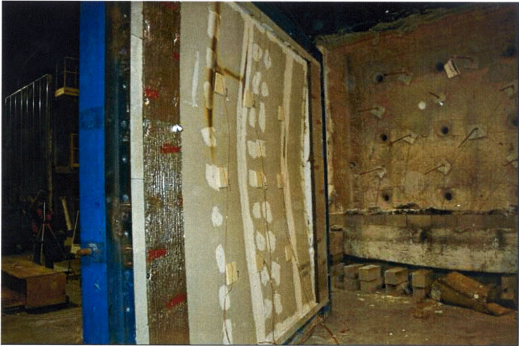
Figure B-10. Unexposed Side of Wall Assembly After the Fire Test.
