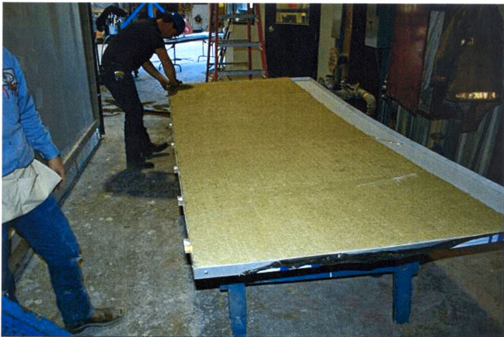
Figure B-4. ACP Panel Insulation in Progress.
