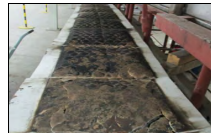
Core after the test (located near the fire end)
