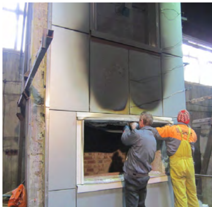
ALUBOND PANELS – REMOVED FROM WALL ASSEMBLY
